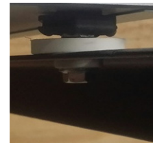
Mounts on rubber grommets to stop vibration
