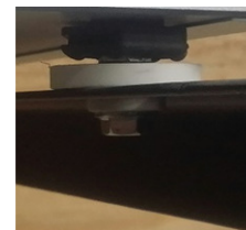
Mounts on rubber grommets to stop vibration
