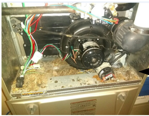
Mice in furnace from a Concentric Vent
